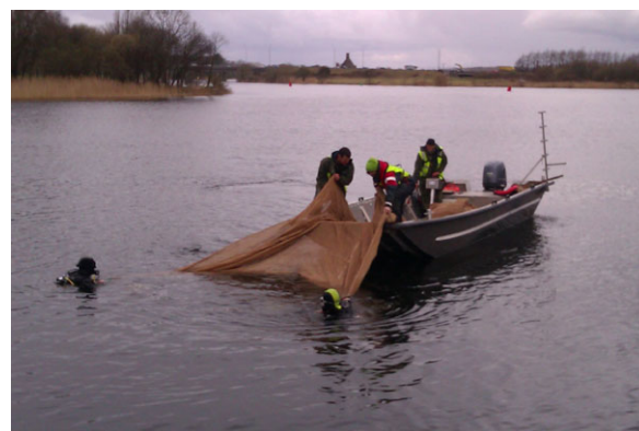
Fig. A5 Application of a geotextile at the bottom of a lake in Ireland to manage Lagarosiphon major . © Johan Van Valkenburg, Dutch NPPO.
