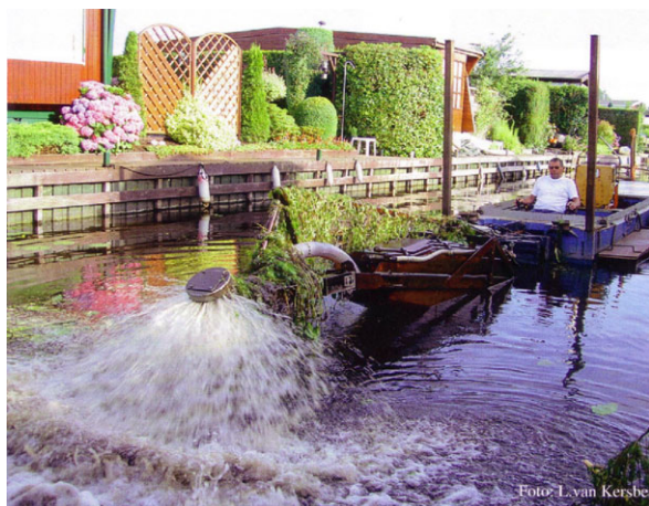
Fig. A3 Dredging using a powerful water-jet in the Netherlands. On the picture, the water jet is raised above water to illustrate its operation. © L van Kersbergen.
